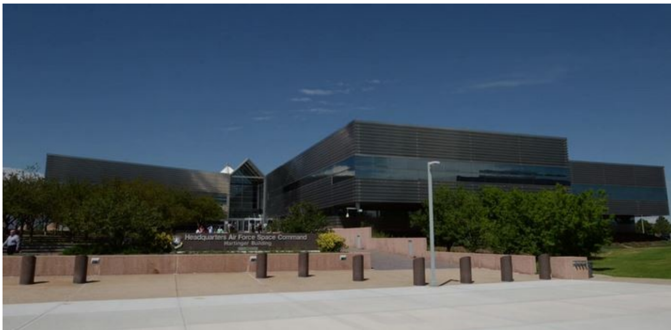
Figure 1. Headquarters - Air Force Space Command, Peterson Air Force Base. Note that google.com/maps shows a different building and different location for the headquarters. (who would alter information on google maps?)
