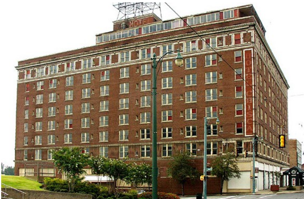
Figure 1. Vacant Hotel Building
