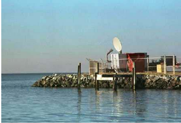
F13. In our ground based system, the principal system elements are a power supply, a modulator, an HEM source, and an antenna. These components are supported by control and cooling systems. The power supply and operators' console(s) are housed in a shelter mounted on one flatbed trailer while the remaining components are mounted on a second trailer (out of the field-of-view to the right). The system is designed to broadcast 2 MW peak power pulses with an average power of 300 kW for 30-second missions. This yields a peak fluence of 1 mW/cm 2 at 2400 ms range.
